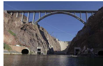
Hoover Dam Bridge
