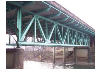
Under Truss Bridge
