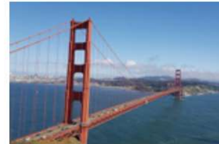
Golden Gate Bridge, California
