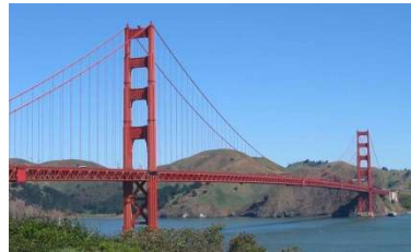
Golden Gate Bridge San Francisco
