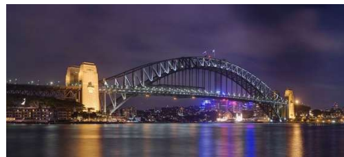
Sydney Harbor Bridge
